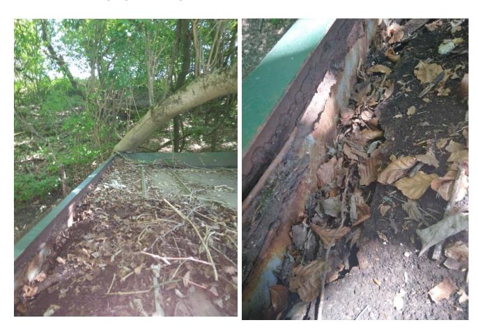
**Item 1** – The roof has corroded and is no longer watertight. The tree is growing around the structure exerting force onto the building.
