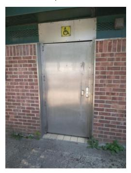
**Item 3** – The brickwork is also distorting at the top and the door no longer closes in this corner. Also, you can see the gaps at the tops of the door, how uneven the building is.
